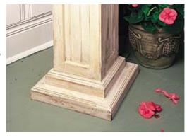
and nail and glue them around the column where it attaches to the base. This detail will add decorative interest and visual weight to the base to keep it from looking top-heav.
