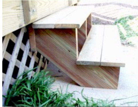
Stairs with 3 risers at 8 1/4" each
