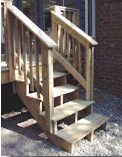
Stairs with 5 risers at 7" each
