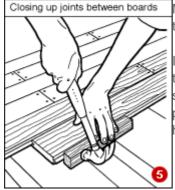
Make sure that the tongued and grooved joints are well seated together before fixing panels to the joists (5).
