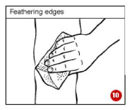
Apply further jointing compound to fill the tape and allow to set. Now apply a final thin coat and feather out to just beyond the tape, smoothing it with a damp sponge just before it sets (10). Allow to dry and lightly sand to remove any high spots. Apply a drywall primer to the entire surface of the board and joints before final decoration.
