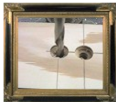
Drilling the Bolt Hole
