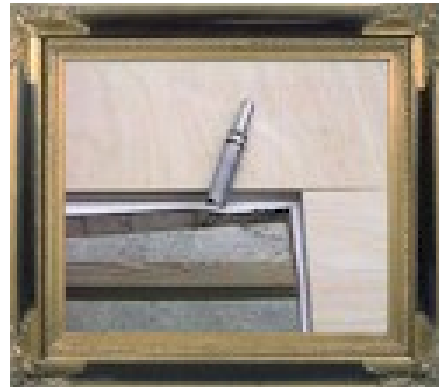
Trimming the Hole
