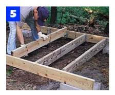
Lay the front and rear joists on the corner blocks. Then, cut the joists, position them in the joist hangers and secure with nails.
