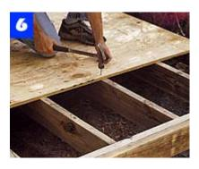
After doubling the front and rear joists, add the 3/4-in. plywood floor. Nail it in place with 8d nails spaced about 6 in. apart.
