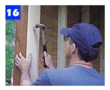
Cut stock for doorjambs and nail in place. At a window, install the angled sill piece first, then the top jamb, then side jambs.
