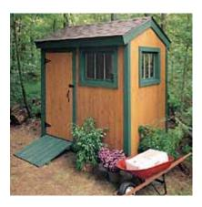
Solid framing, plywood sheathing and cedar siding make this a shed to stand the test of time. Our 6 x 8-ft. design is expandable to 8 x 12 ft.
