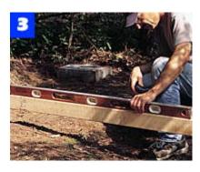
Use a straight 2 x 4 and a 4-ft. level to check that the corner blocks are installed at the same height.
