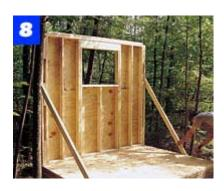
Install 1/2-in. plywood wall sheathing on the framed back wall. Then, raise the assembly and secure it with diagonal braces.
