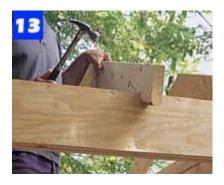
With all the rafters assembled in pairs, position each pair on the wall top plates and secure by toenailing.
