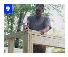
Frame and raise the remaining walls without sheathing. After nailing together the corner studs, add the top plates.
