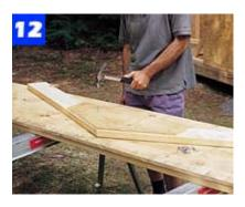
Set up a worktable with the outline of the rafter assembly marked. Then, join each pair of rafters with a plywood gusset.
