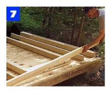
With the back wall framing members cut to length and headers assembled, lay out the pieces on the shed floor and join with nails. Stand the rear wall, bracing it with 2 x 4s nailed between the wall and the outside floor joists (Photo 8). Nail the bottom plate to the deck so the plywood sheathing is flush with the edge of the deck.
