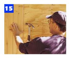
Nail 1 x 6 tongue-and-groove cedar siding in place. Use 8d nails over wall framing and 6d nails when nailing into plywood alone.
