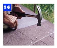
Use 1/2-in. plywood for the roof deck and cover it with roofing felt. Install shingles following the manufacturer's instructions.
