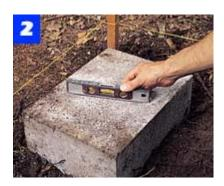
Dig a hole for the first block at the highest point in the grade. Add gravel, install the block, align it with the string, and level it.
