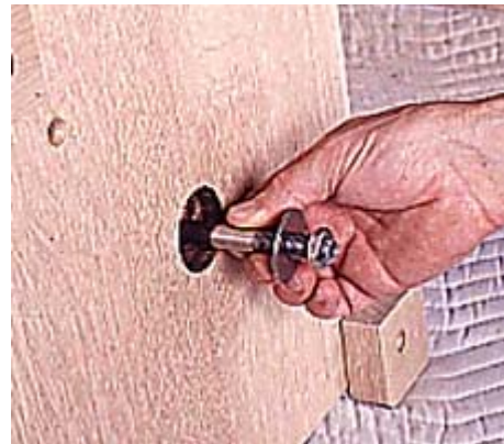
9--Install a washer and nut on one end of the steel pipe, then slide it into the post's hole. Adjust the height by turning the nut.
